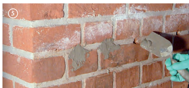
Closing of drill holes
