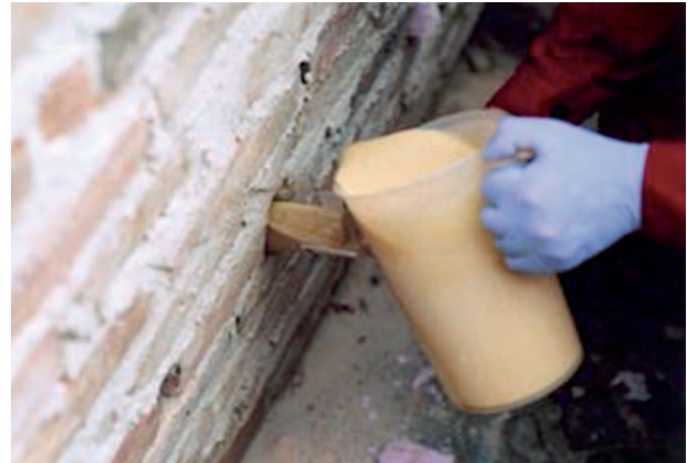
Application of WEBAC. 2260
