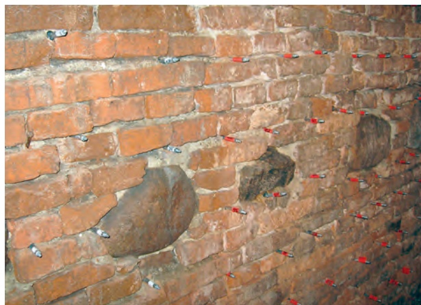
Filling of cavities/voids
