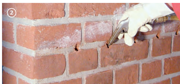
Extraction of drill dust
