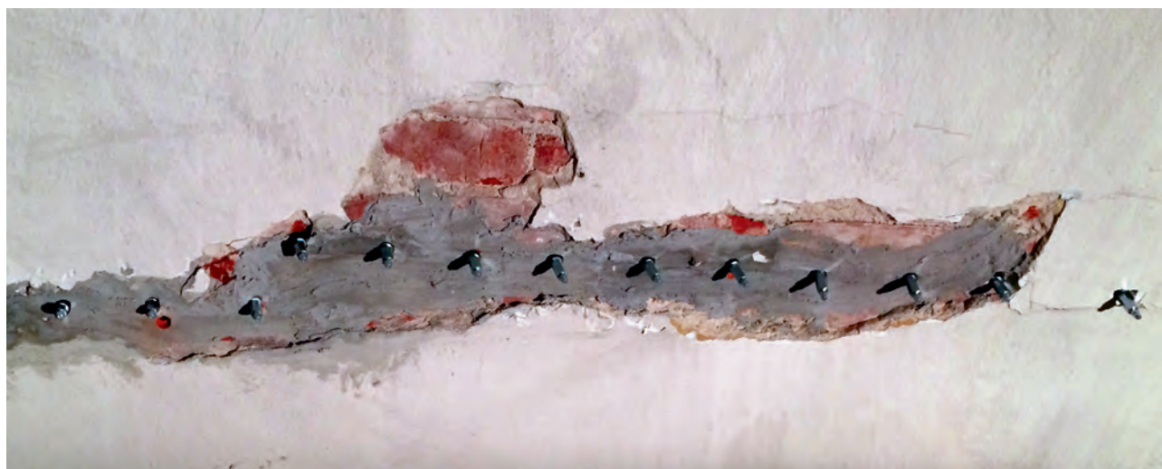
Positioning of packers
