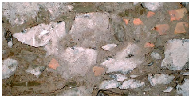
Natural brickwork with loam mortar joints
