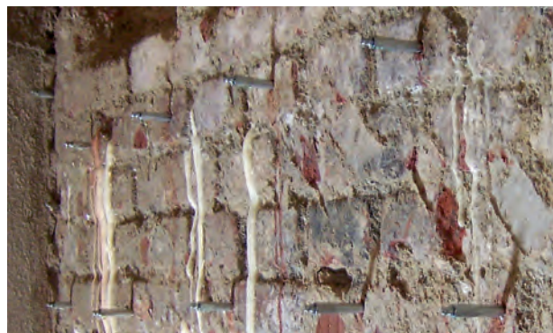
Filling of cavities/voids
