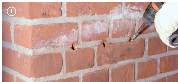
Making of drill holes (masonry size 24 cm)
