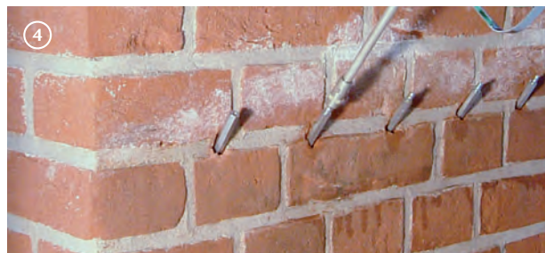
Injection of PU injection resin
