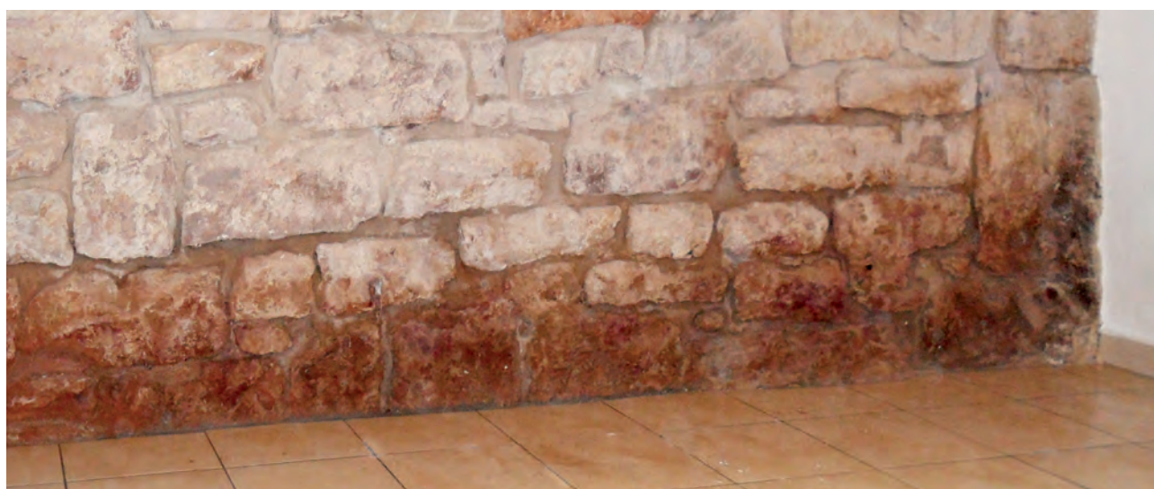
Moisture-damaged masonry
