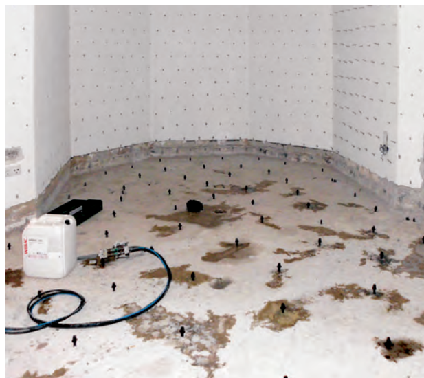
Positioning of packers in wall and floor area
