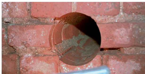
Core removal from brickwork
