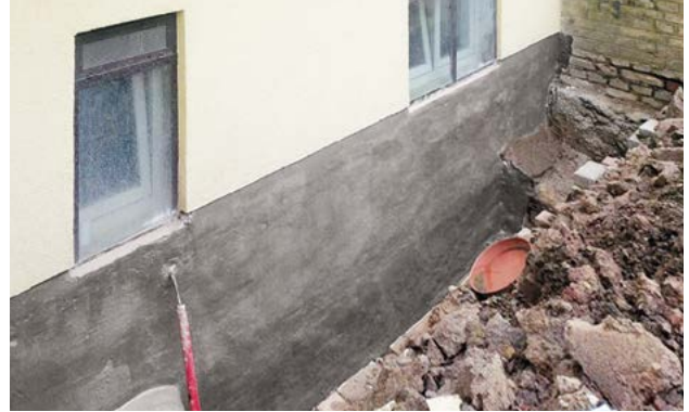
Fig. 2: Prepared substrate
