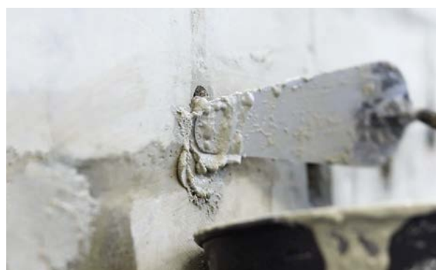
Fig. 6: Closing drill holes
