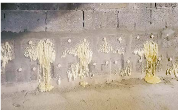
Fig. 5: Filled hollow block
