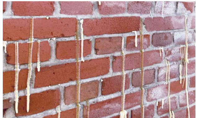
Fig. 4: Material discharge
