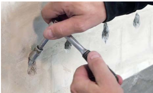
Fig. 3: Screwing in packers
