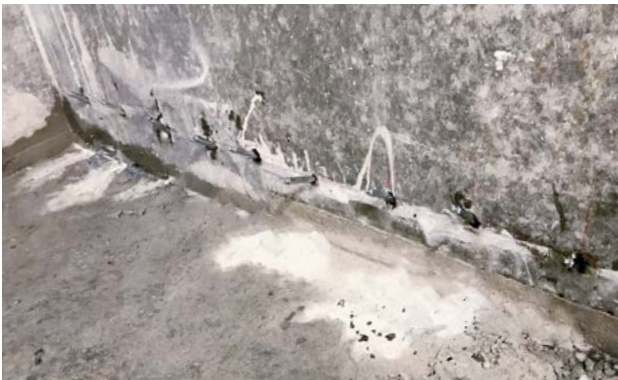
Fig. 3: Setting the packers
