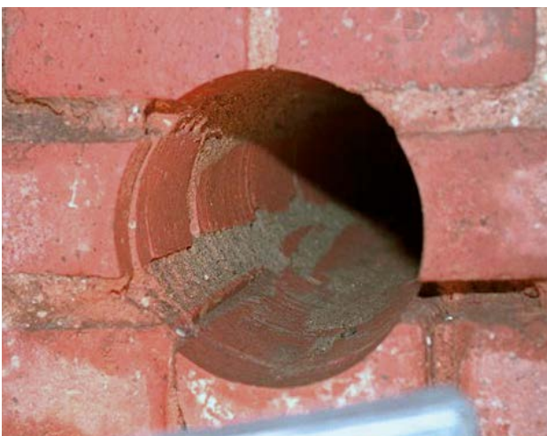
Core sampling on the building component
