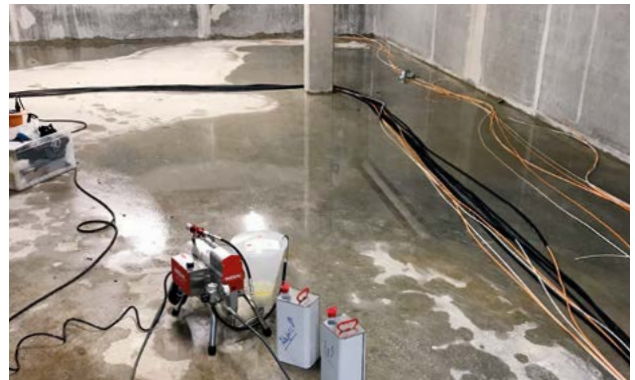
Fig. 4: Injection of wall-floor joint
