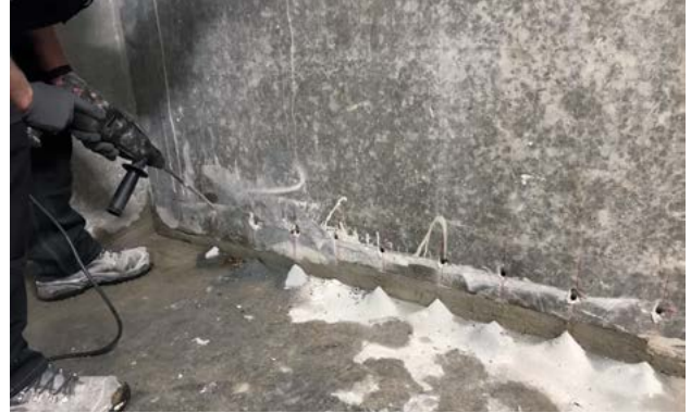
Fig. 2: Drilling the drill holes
