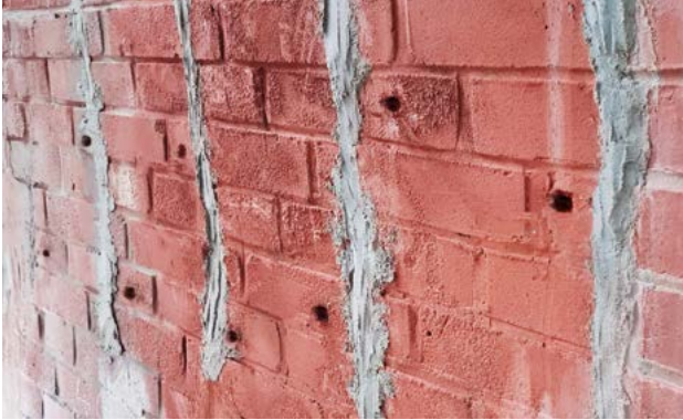
Fig. 1: Drilling and cleaning holes
