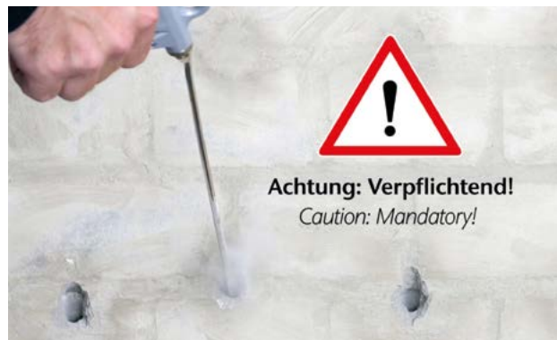
Fig. 2: Extraction of drill dust
