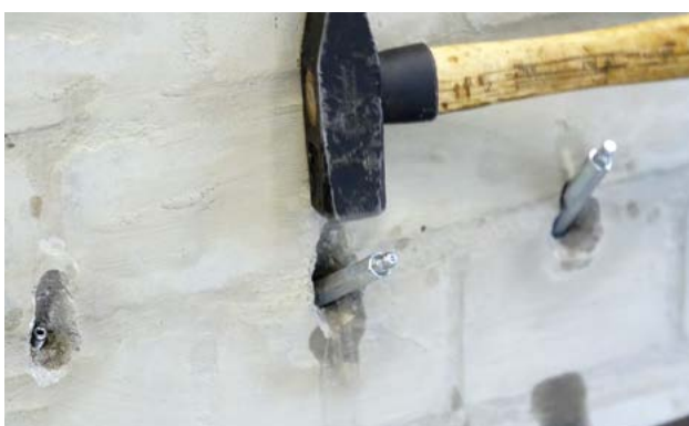
Fig. 5: Knocking out packers
