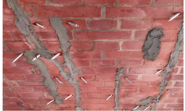
Fig. 2: Setting packers
