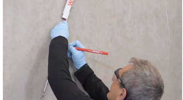
Fig. 2: Determining the surface packer spacing above the crack
