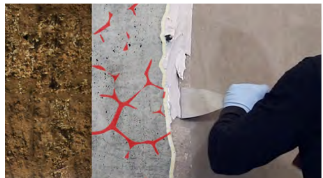
Fig. 6: Removing the patching and packers
