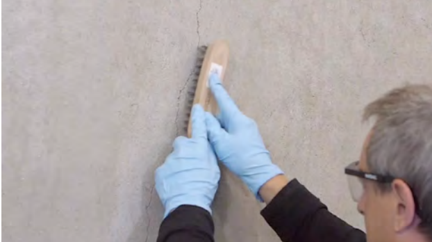
Fig. 1: Cleaning of the surface
