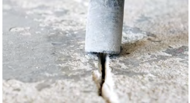
Fig. 2: Remove dust completely
