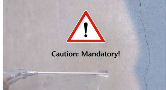
Fig. 2: Removing drill dust
