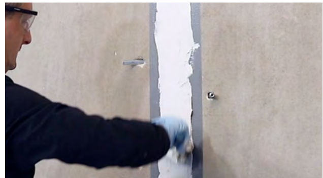
Fig. 4: Patching of cracks
