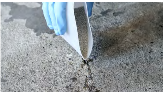
Fig. 5: Filling of the crack after impregnation with quartz sand
