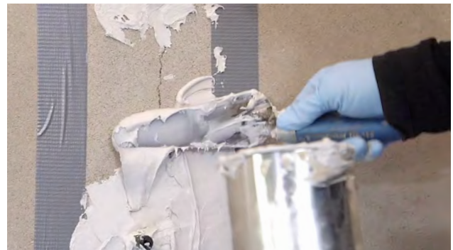
Fig. 4: Patching and gluing of the surface packers
