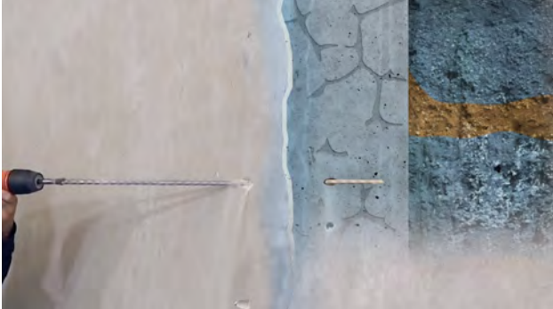
Fig. 1: Making drill holes
