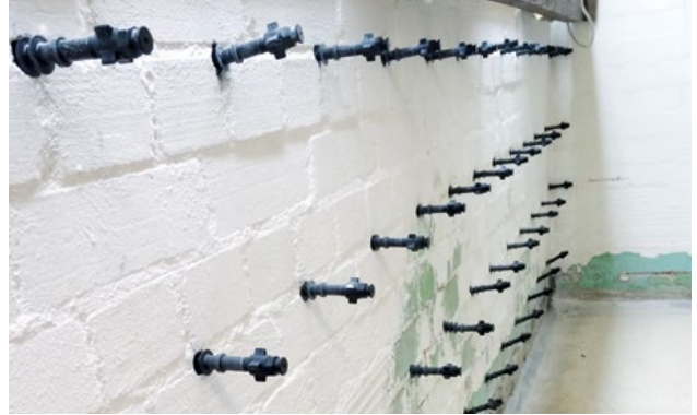
Fig. 2: Example of packer positioning
