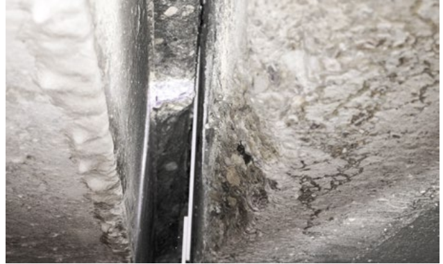
Fig. 2: Clearing joint, cleaning joint edges, cutting open joints if necessary
