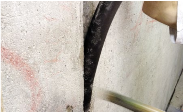
Fig. 3: Installing hammer-in profile
