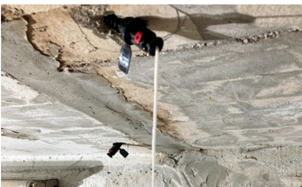
Fig. 5: Injecting material
