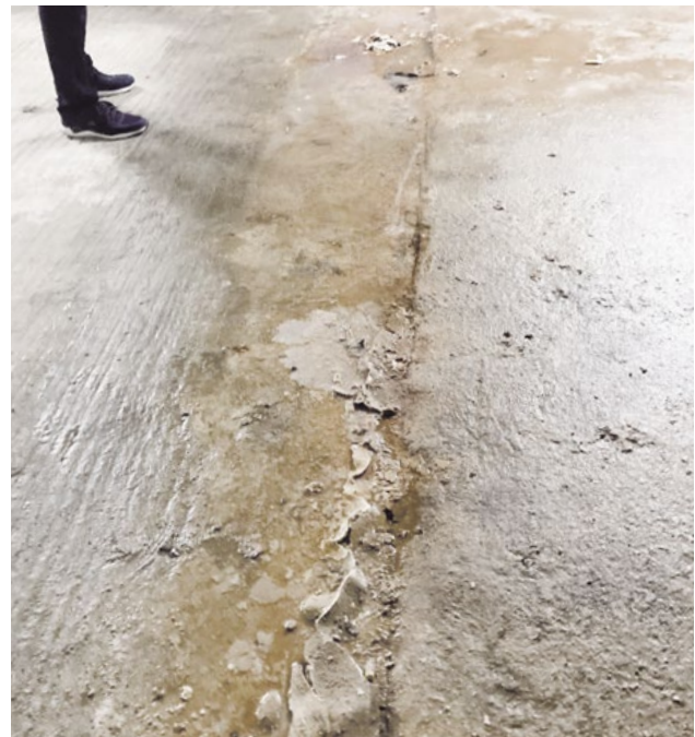
State of construction before renovation
