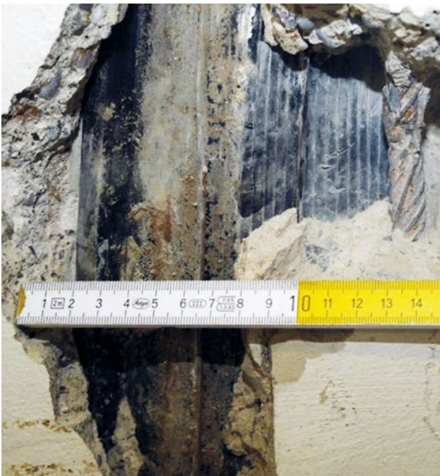
Measurement of a brittle expansion joint
