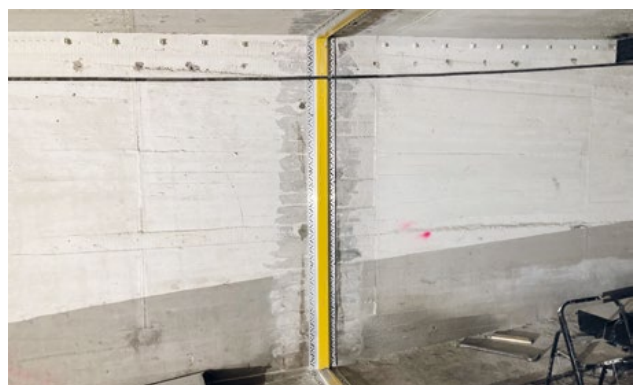
Fig. 6: Reworking joint
