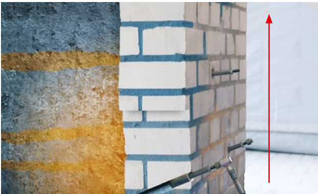
Fig. 3: Injection from bottom to top
