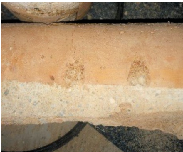
Drill core removal
