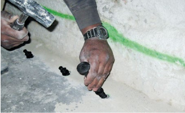
Fig. 1: Marking the drill hole grid, drill holes and place packers
