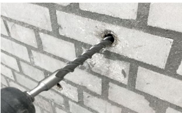
Fig. 5: Removing packers – drilling out (at least 10 cm) and sealing drill holes
