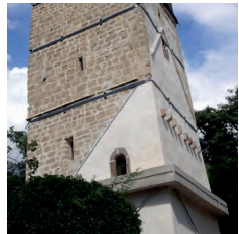
New gypsum render on the inclined wall surface
