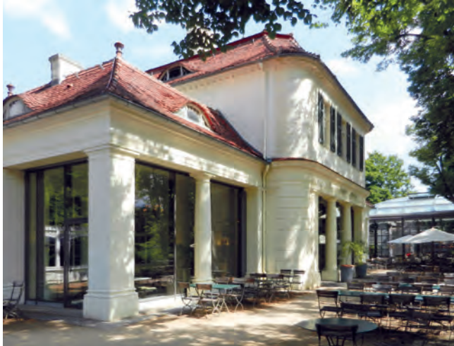
Also almost 20 years after its renovation the building looks sparkling new
