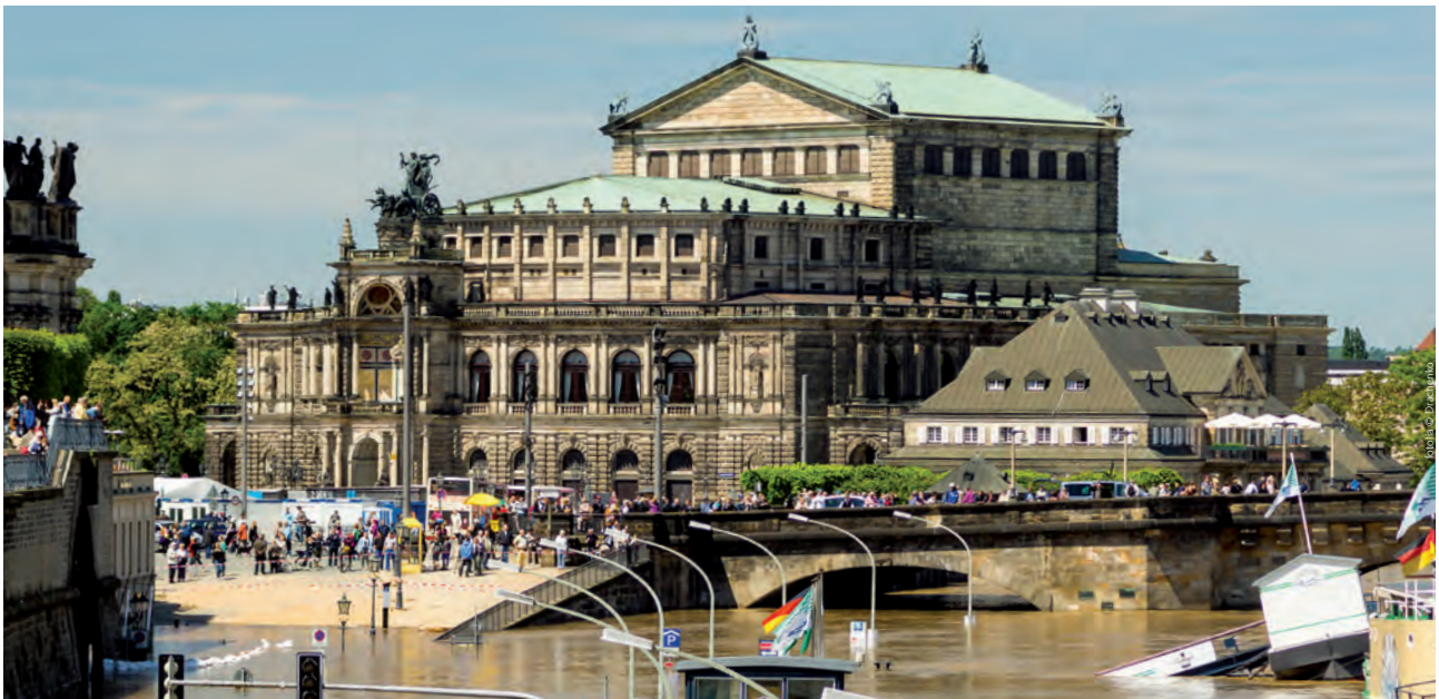
Semper Opera House in Dresden during River Elbe flood in 2013
