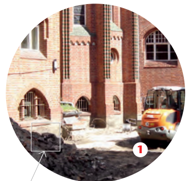
during the construction work in the town hall courtyard
