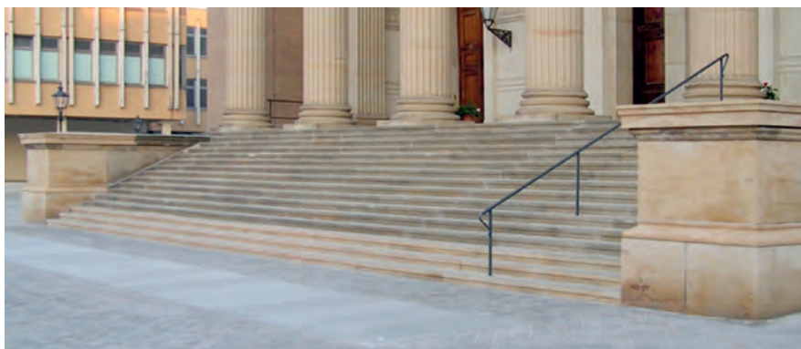
Freshly restored natural stone stairs
