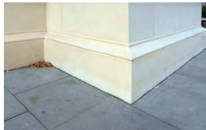
Permanent sealing of plinths against surface water
