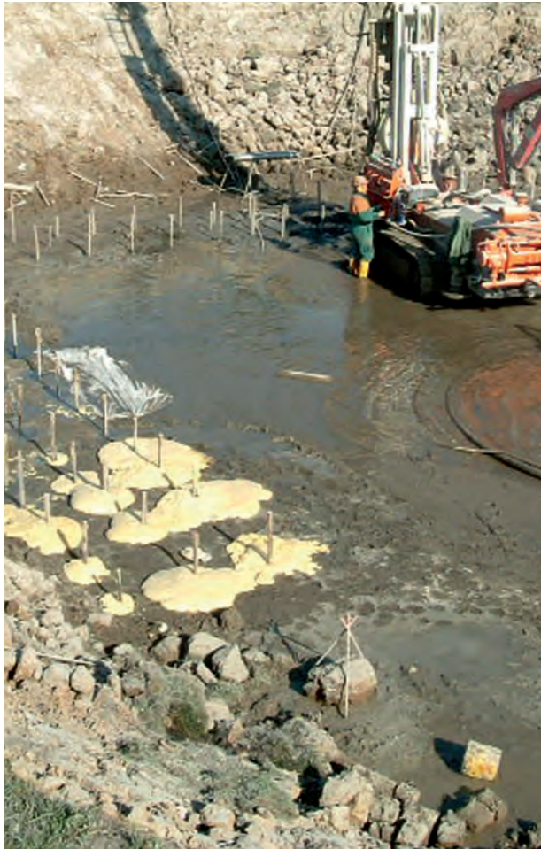
Application of WEBAC polyurethane foam resins
